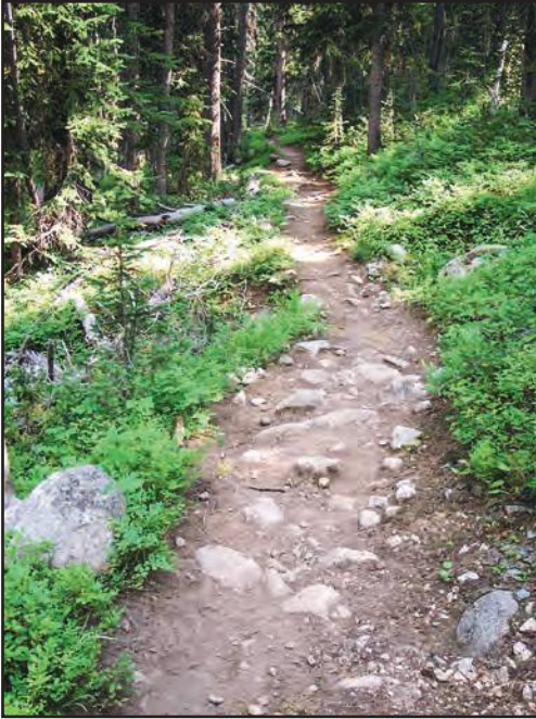
Trail Class 3: Tread —The tread is continuous and obvious.
