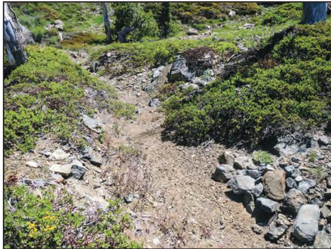
Trail Class 2: Obstacles —Obstacles may be common and substantial. Blockages are cleared to define the route and protect resources. Vegetation may encroach into the trailway.
