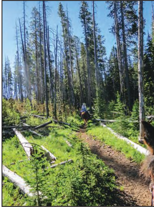
Trail Class 3: Tread —The tread is continuous and obvious.
