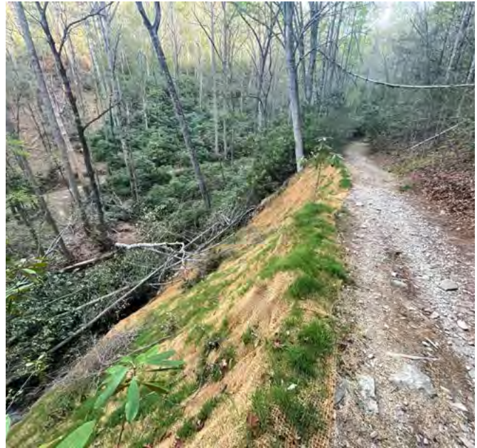
After a slide on Thrift Cove, the trail's exposed, disturbed soil and frequent foot traffic created ideal conditions for invasive plants to take hold. Field staff stabilized and reseeded the slide to reduce erosion and help establish native vegetation.
